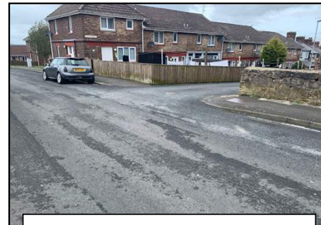
Site Photo – taken Victoria Road April 2024
