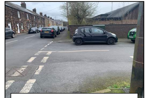
Site Photo – taken Spencer Street April 2024
